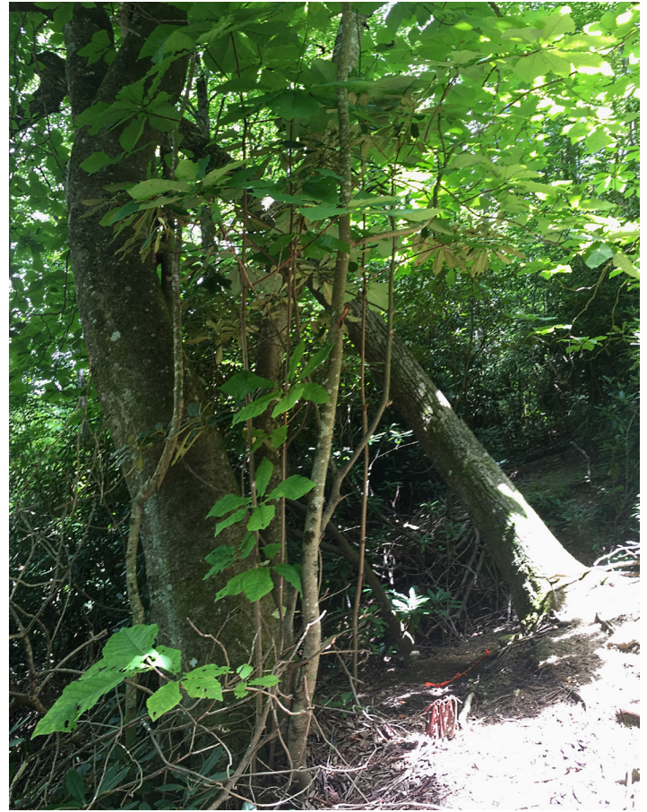
Figure 8. Photograph of curved and leaning trees on the rock slide. Slide movement is downhill toward the left (north). 2018_07_05 NCGS photo.
