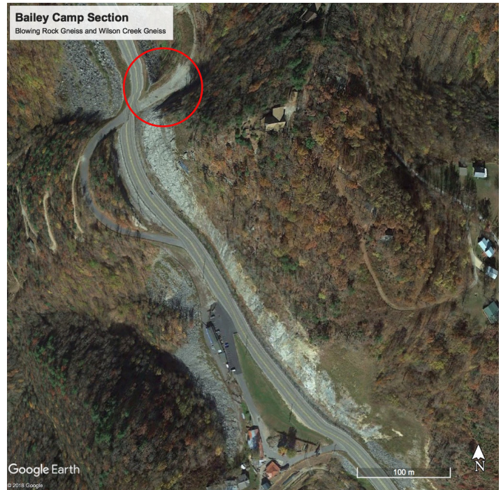
Figure 2. Bailey Camp section. Gravel parking lot indicated by red circle.
