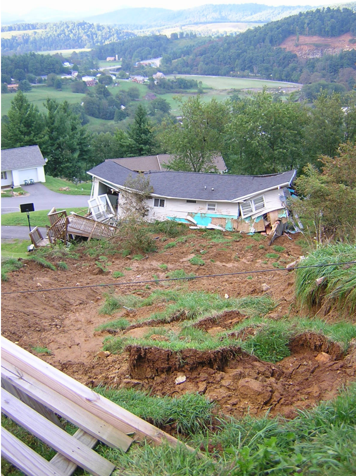
Figure 5: Home in the White Laurel community destroyed by an embankment (fill) failure that mobilized into a debris flow on September 8, 2004 during rainfall from the remnants of Hurricane Frances. 2004/09/08 NCGS photo.
