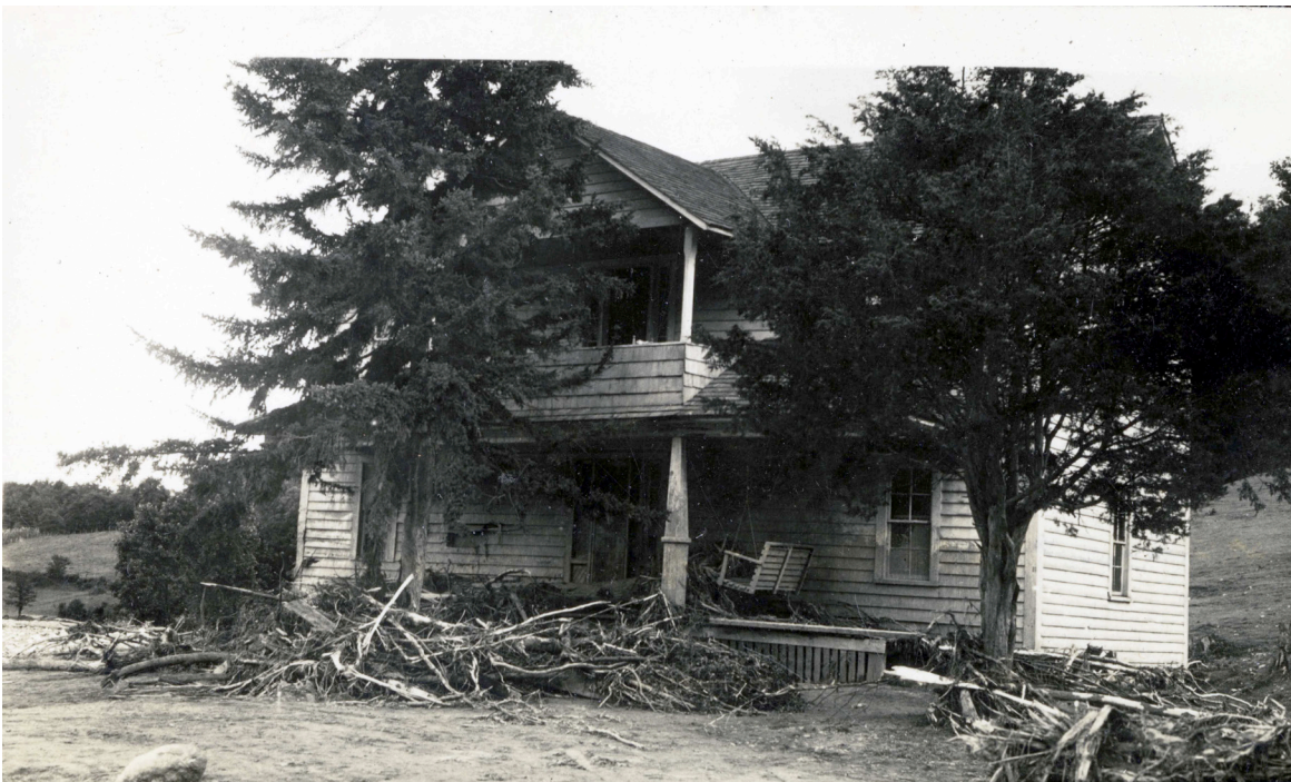
Figure 2: Photograph of the home of Zeb Greene taken soon after the 1940 flood. The cedar tree on the left is probably the tree that saved Worth Greene’s life that night, based on the direction of flow. Also, notice the prominent mud line on the front of the building and porch posts, indicating the height of the debris flow as it surged past the house. (Source: Paul Weston, “Zeb Greene House, Stony Fork, August 1940,” Digital Watauga, accessed August 16, 2018, https://digitalwatauga.org/items/show/6368 .)
