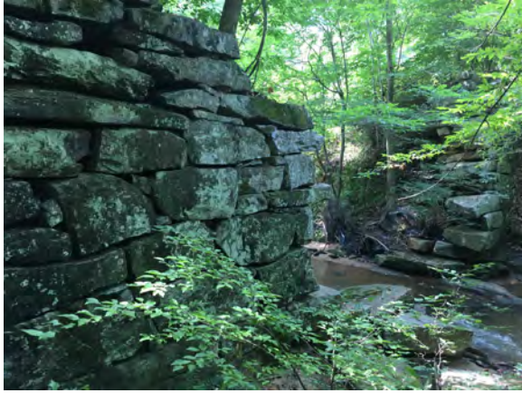
FIGURE 9: The former Richmond Mill Pond dam at Stop 1.6 was constructed with slabs of Connally Church orthogneiss.
