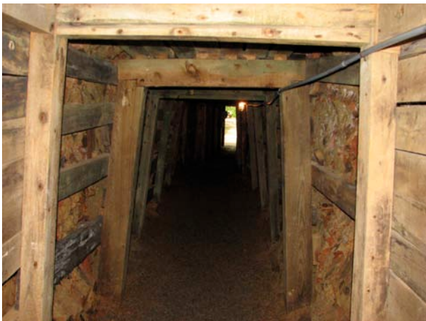
Figure 24. View from inside Linker adit at station 3 looking towards the entrance.
