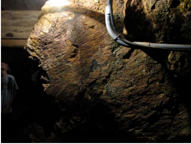
Figure 26. Slickenlines at interface between greenstone and quartz vein (removed), at light by station 7. The oblique orientation of these features on the vein margin is consistent with sinistral reverse motion in the Gold Hill shear zone.
