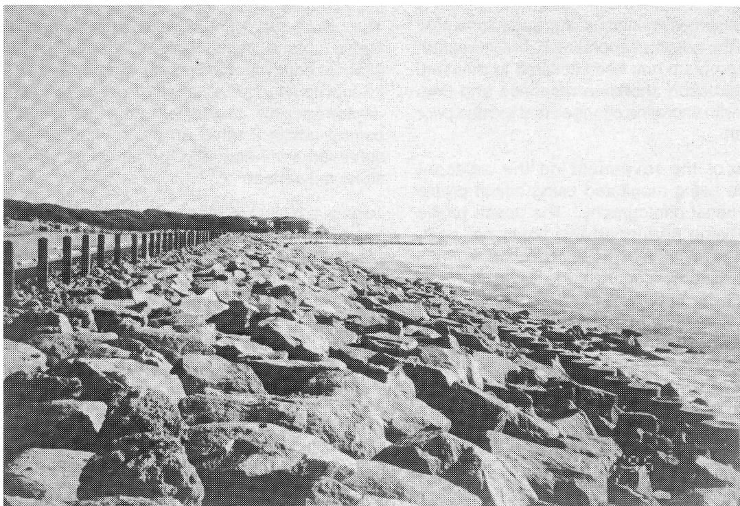
Figure 5. View of completed revetment looking northward from the Battle Acre area.
