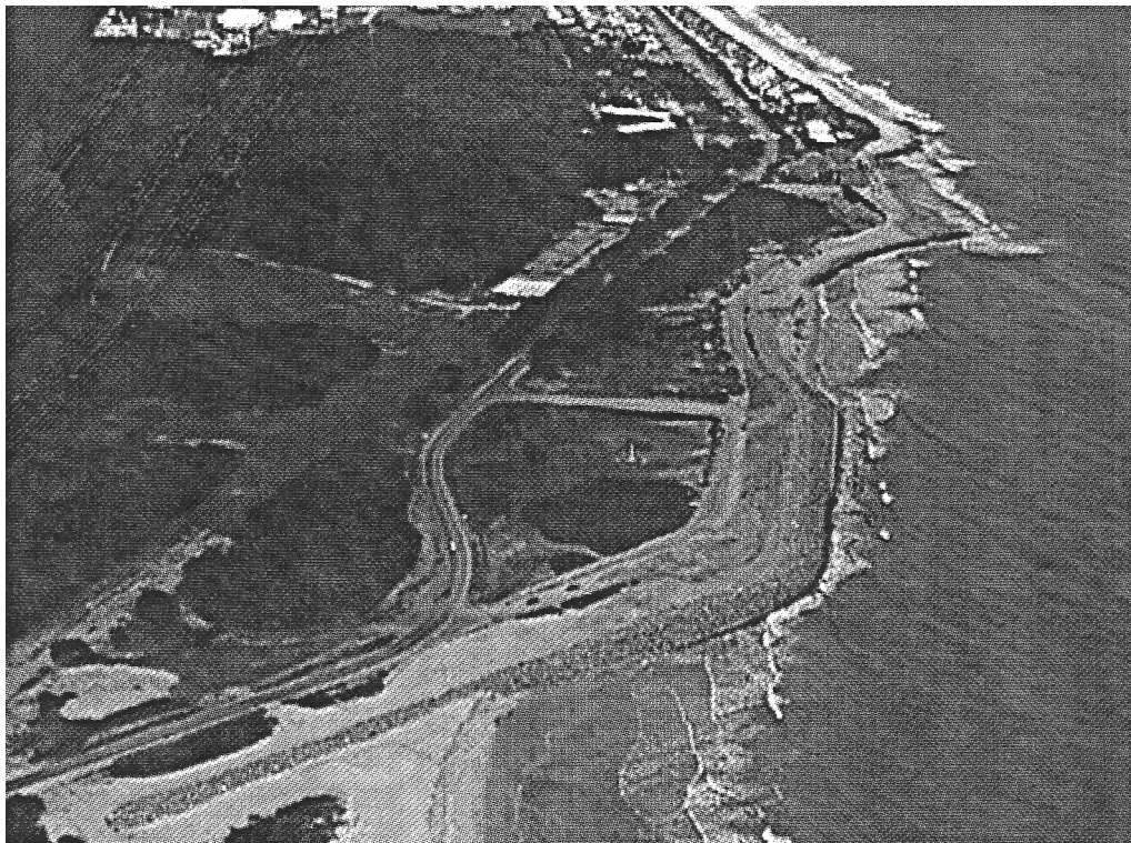
Figure 39. Fort Fisher Seawall. Aerial Photograph (1996). The 3,050 ft long revetment completed in early 1996, was a controversial issue which required a variance and special permit. Crestal elevations range from 10 to 16.5 ft. The 70 foot wide base is fronted by huge 5 ton interlocking pods. The structure fared reasonably well during Hurricane Bertha and suffered minor damage during Hurricane Fran.
